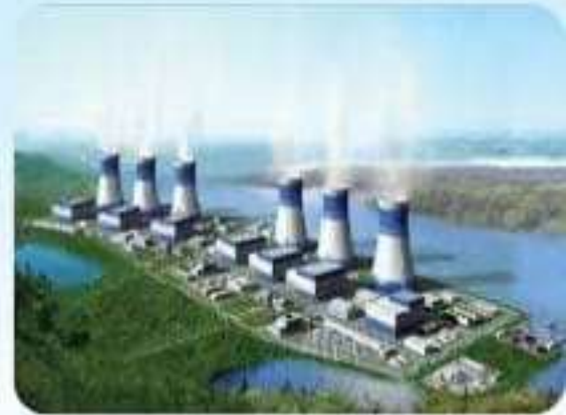
Nuclear power plant
